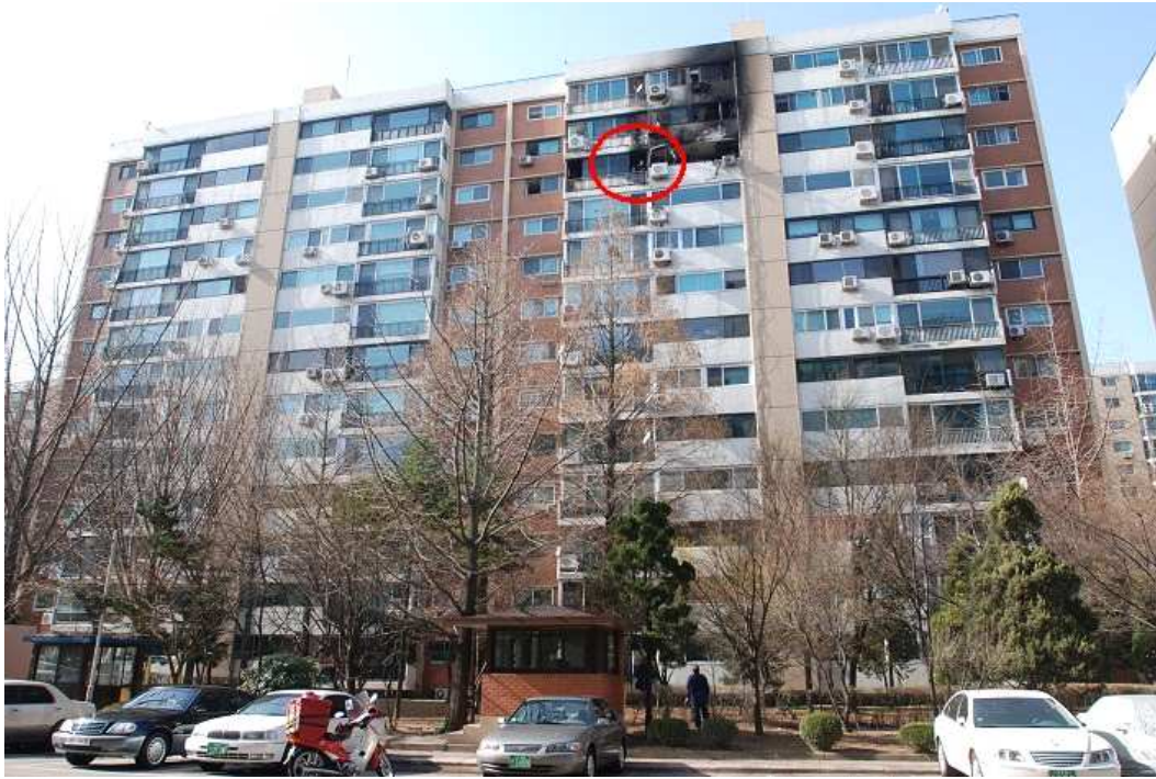
<Photo 3> View of the apartment (area encircled in red indicates the location of the fall)
