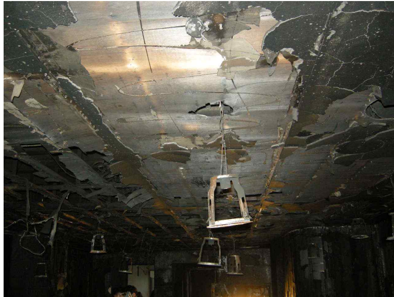
<Photo 9> Ceiling inside the room
