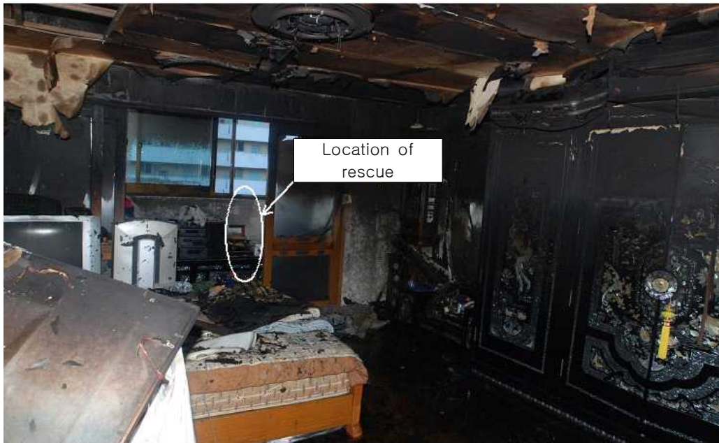
<Photo 6> Inside the main room
